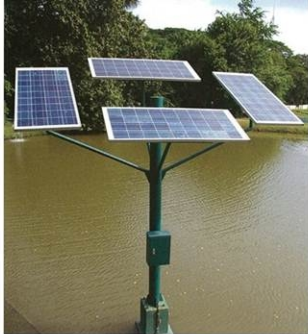
Solar panels generating electricity for pumping water
